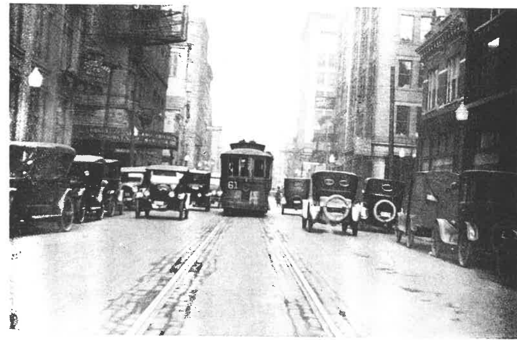
SIMILAR DOWNTOWN STREET BUT WITH ONE CAR TRACK Two clear moving traffic lanes outside of car tracks
