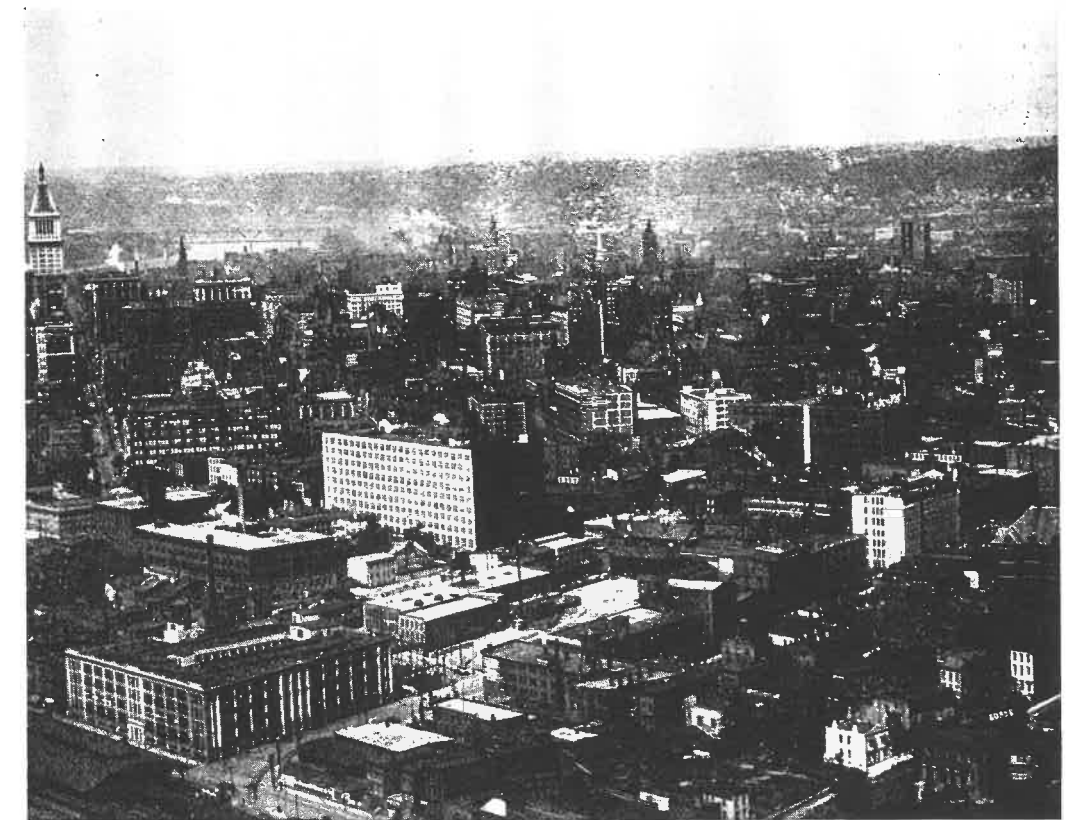
THE "BASIN" FROM THE SOUTHEAST
