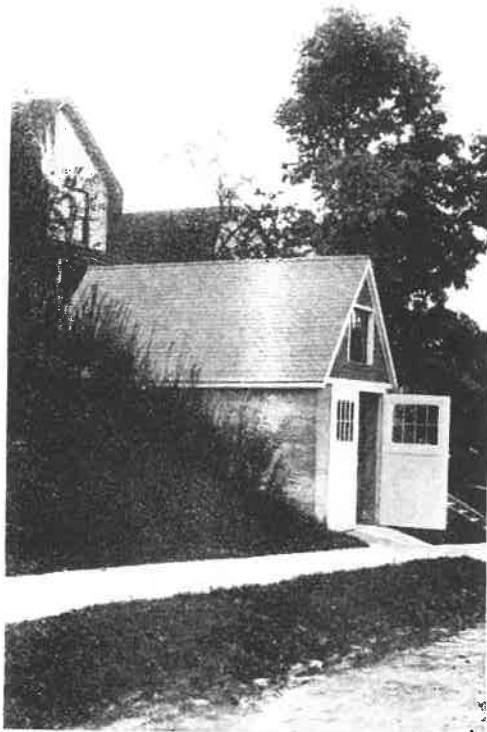
A PRIVATE GARAGE SPOILING A HOME STREET. Doors swing over street and garage masks houses.
