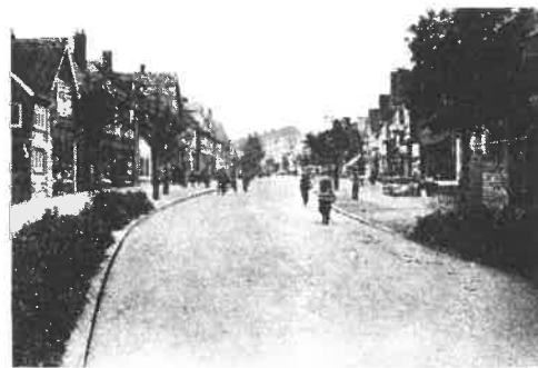
LETCHWORTH, ENGLAND MAIN BUSINESS STREET Note trees, setback and harmonious treatment of fronts
