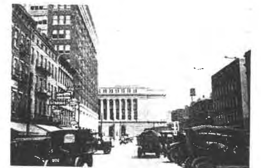
COURT STREET TOWARD COURT HOUSE AFTER WIDENING One half of facade visible
