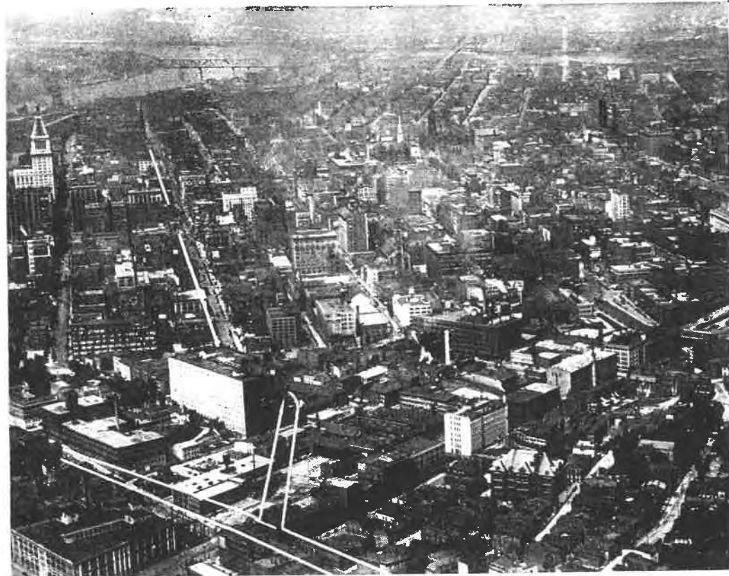
WHOLE "BASIN" FROM EAST Aeroplane view of Third and Fifth Street improvements
