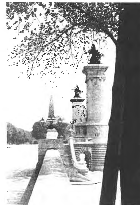
PARIS, APPROACH TO THE ALEXANDER III BRIDGE A striking bridge entrance
