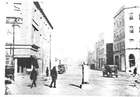
BANK STREET, NORFOLK, VA. Street recently widened twenty feet on the right side, by property owners agreeing to give land, provided the city would pay the cost of setting back the facades.
