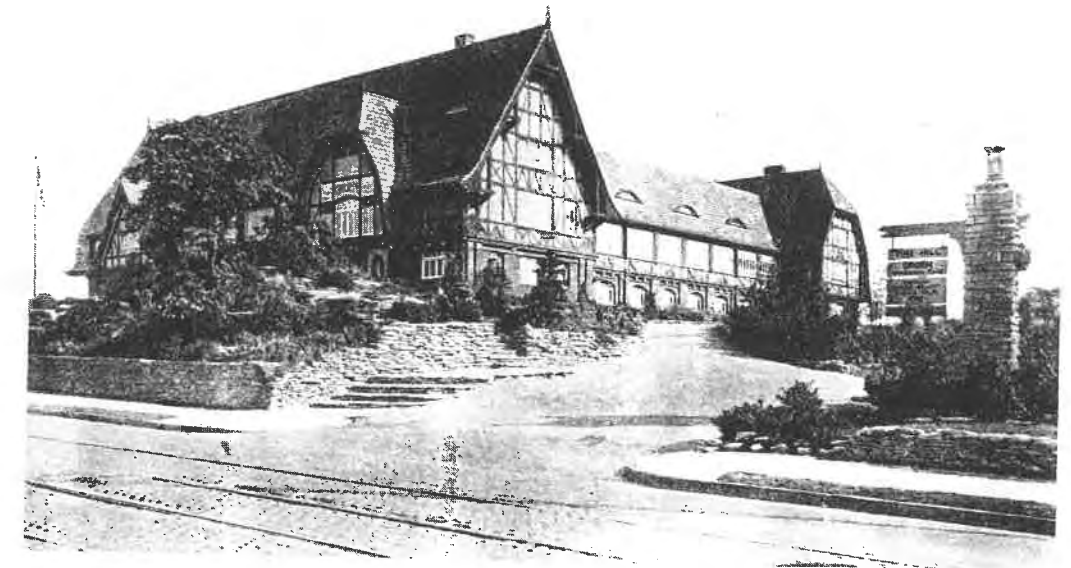
A HILLTOP FACTORY Even a factory can add strongly to the charm of the city
