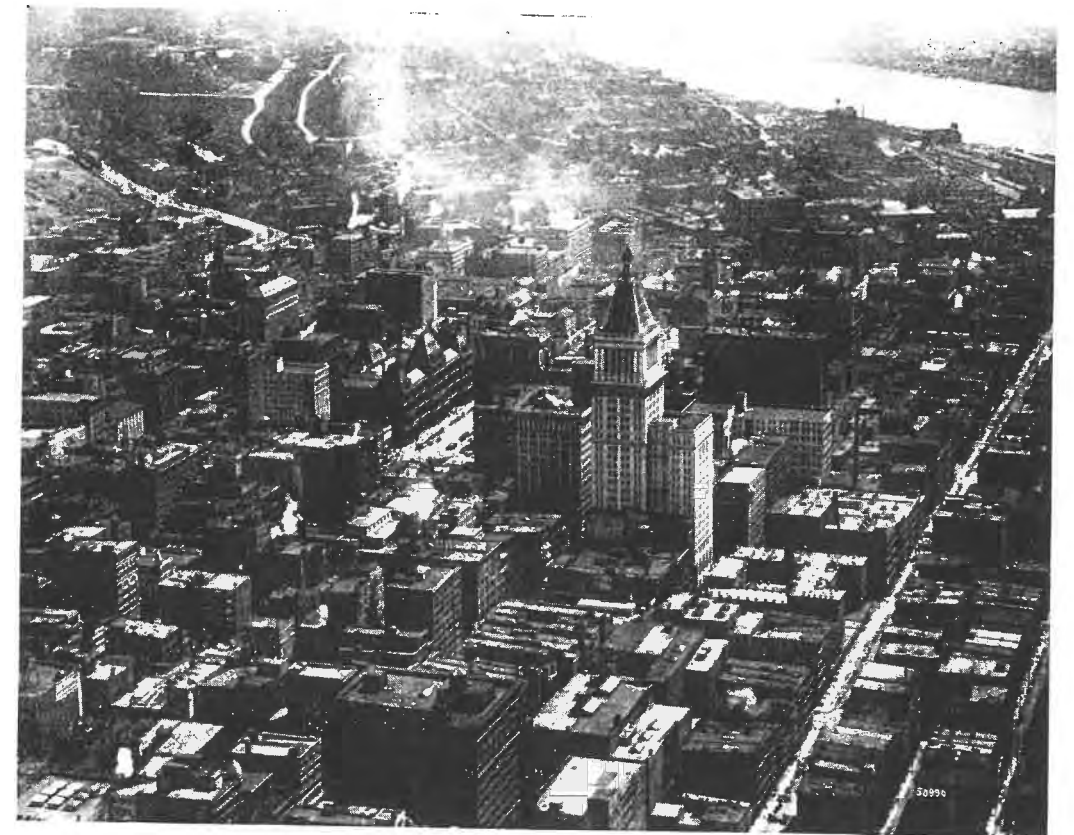
THE "BASIN" FROM THE NORTHWEST — MT. ADAMS IN THE BACKGROUND
