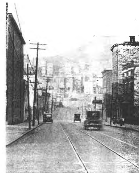
FREEMAN AVENUE TOWARD FAIRVIEW HILLTOP Suggested site for a "Community Center"
